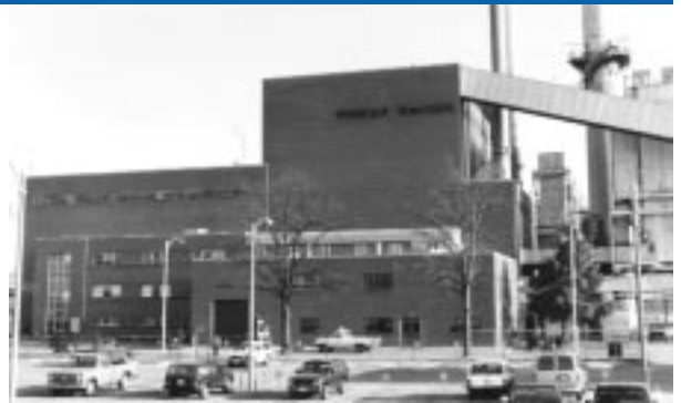
Pictured above is the Blue Valley Power Plant located at 21500 E. Truman Rd.
