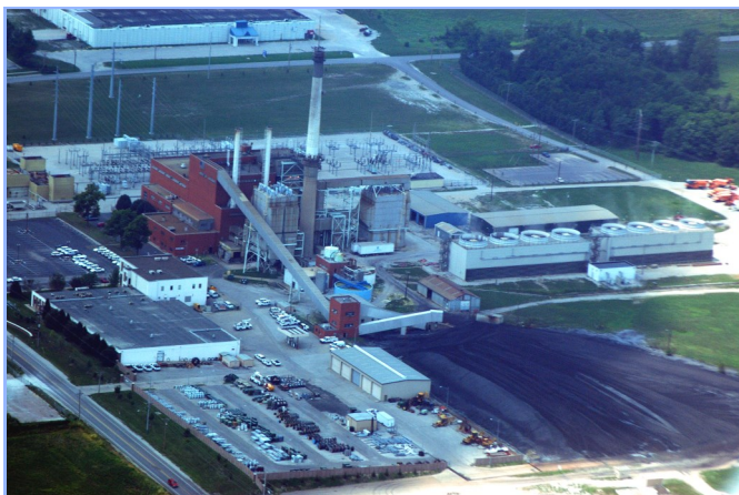
Blue Valley Generator Hydrogen System
