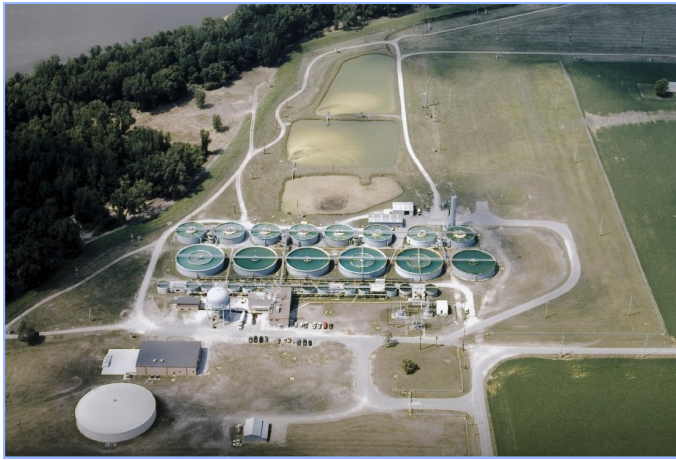
Fiber Optic Connection to Courtney Bend Plant
