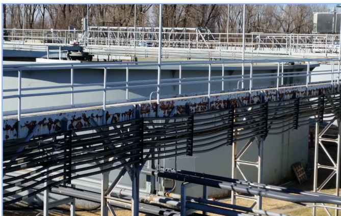
Courtney Bend Water Plant Catwalk Improvements
