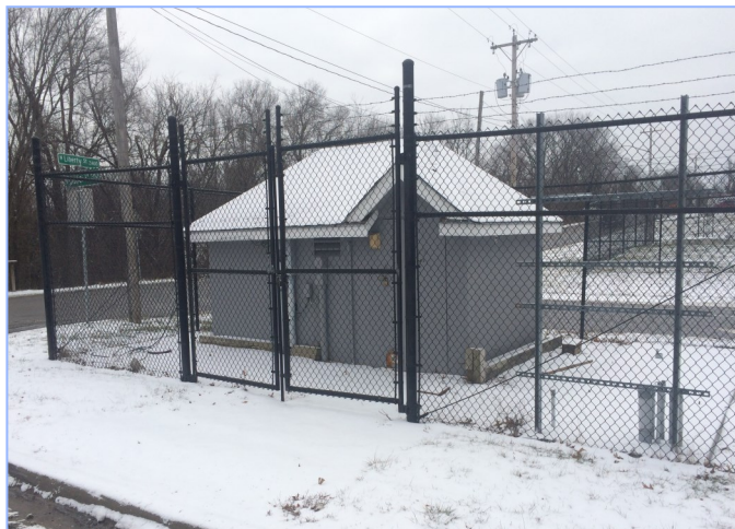
Kentucky 1 Pump Station Demolition
