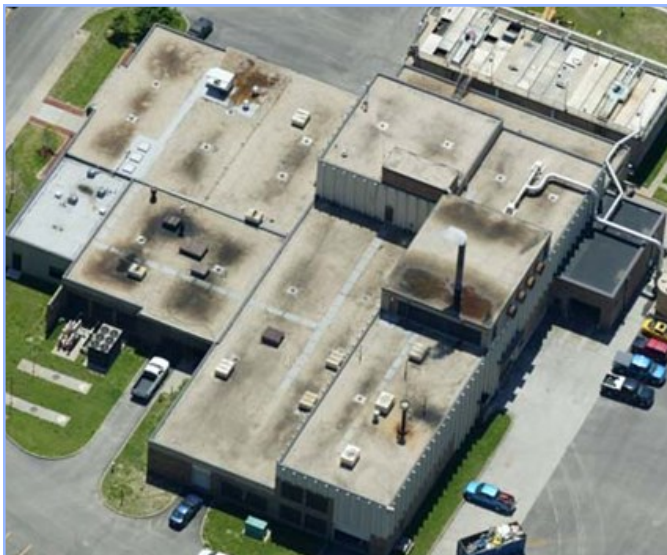
Rock Creek Treatment Facility Project
