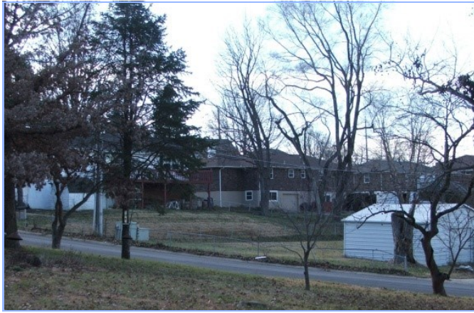
Walnut Gardens Drainage Project
