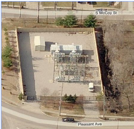
Substation and Transmission Upgrades
