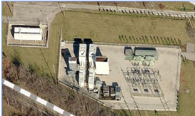
Substation I Transformers & Switchgear Replacement
