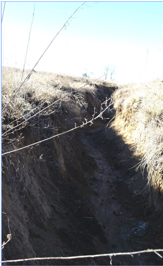
Little Blue Parkway Transmission Main
