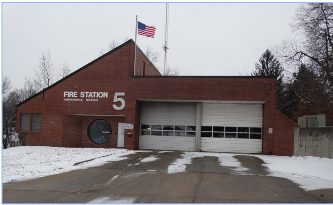
Fire Station 5—Renovation
