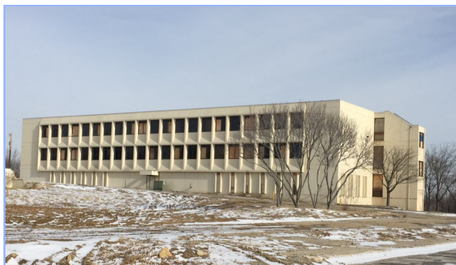
New Administrative Office Building
