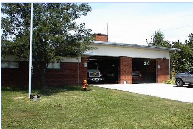
Fire Station 8—Roof Repair
