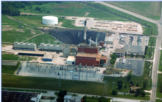
Blue Valley Burner Management System
